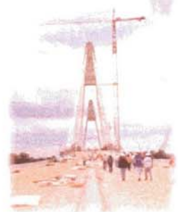
Natcher Bridge under construction. Spring 2001 Photos by: T. Huff
